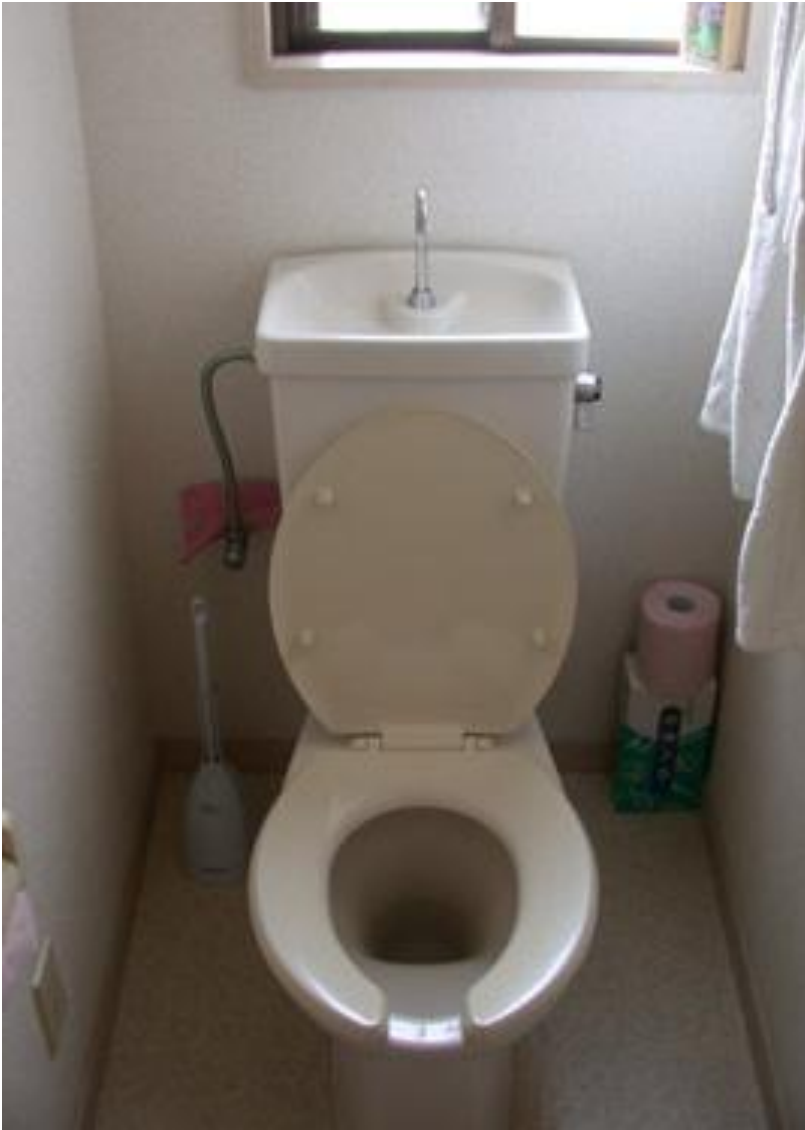
Japanese Toilet – You wash your hands with the water entering the tank, which is then used for the next flush.
