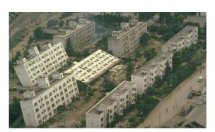
Buildings in the Niigata Prefecture in Japan -An earthquake caused the buildings to fall over because of moisture in the soil.
